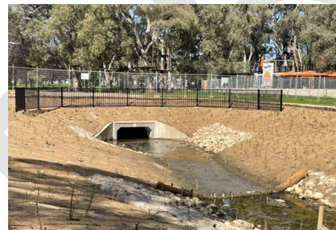
Park 20 new culvert and swale
