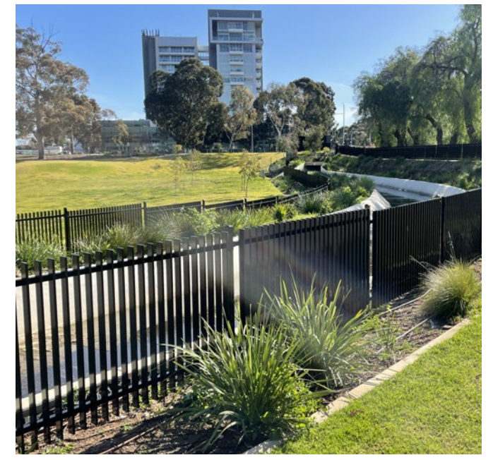
Concrete swale and fencing
