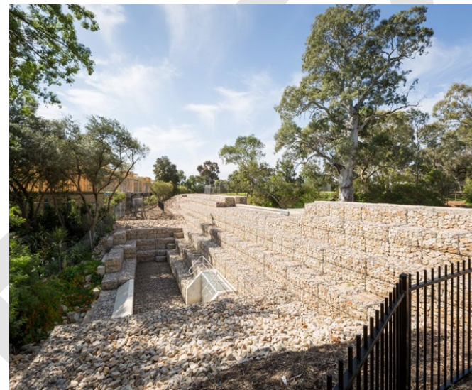
Flood Control Dam
