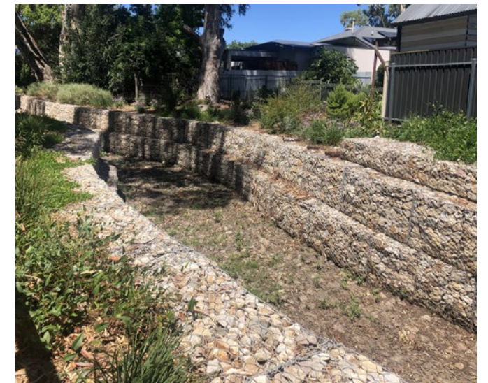
Rock filled gabions
